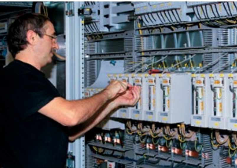
Switch Cabinet Assembly
