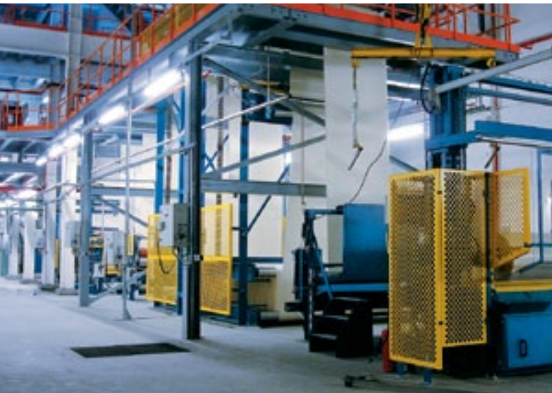
Tire cord installation
